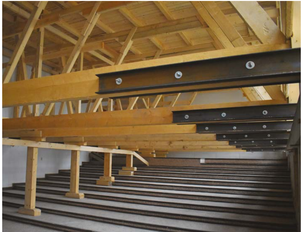
64 | Stabilization of the lecture room No. 034 ceiling during reconstruction (2018)
